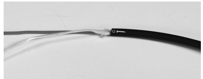
4.3.2 Remove the cable jacket.
