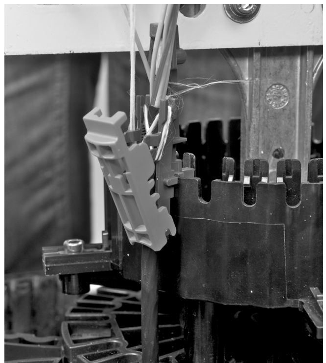
4.3.27 Cut the strength member leaving 2.5cm and install in CTU as shown.
