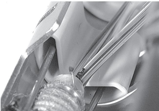
4.2.7 Insert the strength members from the cable into the strength member stop. Secure the cable with the hose clamp onto the loopbracket. Secure the cable with tie wrap onto the loopbracket. Secure the screw of the strength member stop on the loopbracket. Wrap a few layers of tape around the hose clamp.
