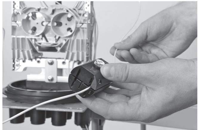
4.1.16 **In case of reversed oscillating cable (SZ-cable):** separate the loose tube(s). Match the loose tube(s) on the tubeholder and mark both sides between the two marks. Shave between the two marks with the appropriate tooling. Clean the fibers and wind some PTFE tape around the ends of the tubes and fibers, to protect the transition from tube to fibers.
