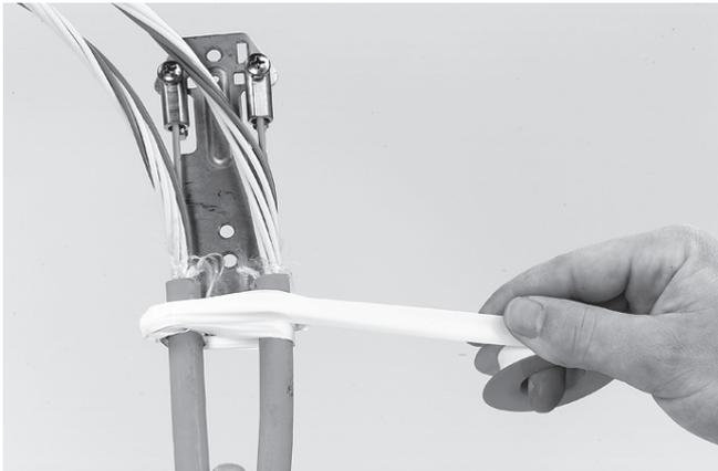
4.1.8 If the cable diameter is more than 8 mm Secure the cables with the hose clamp onto the loop bracket. Wrap a few layers of tape around the hose clamp. If the cable diameter is less than 8 mm secure the cables with tie wraps.
