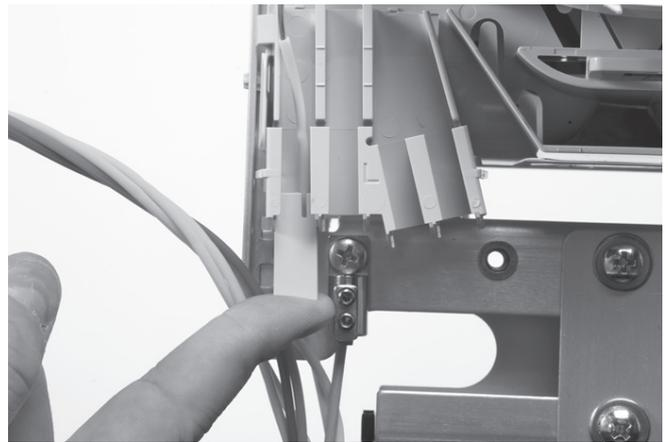
4.1.31 Position one or more loose tubes in the tubeholder according to the correct position and slide the tube holder retainer with the snap forward in the lowest possible cavity of the tubeholder above the loose tube. The tube holder retainer must snap. (see capacity of tubeholders).
