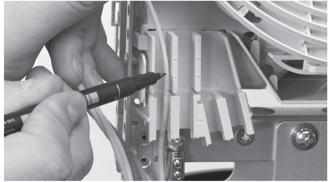
4.1.30 Match the loose tube on the tubeholder, mark and strip the loose tube from this mark. Clean the fibers.
