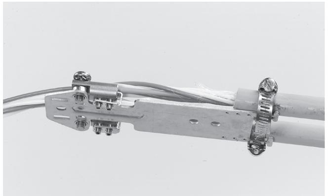
4.1.7 Insert the strength members of the cable into the universal strength member connector on the loop bracket (loosen the bolts with the Allen key if necessary) such that all loose tubes can be routed without unnecessary crossings. Avoid to twist the loop in the case of a reversed oscillating cable. Secure with the Allen key.
