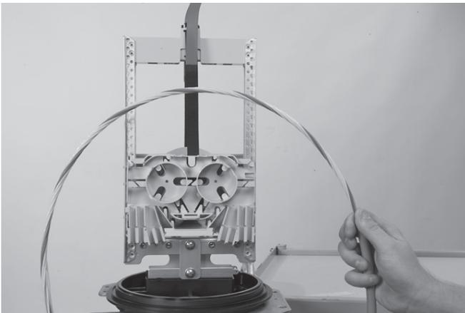
4.1.3 Reversed Oscillating cable: mark the cable in the middle of the loop and remove the cable jacket left and right of the mark over a total distance of 110cm (little more as the distance between two reversal points). Locate the buffer tube reversal point on the cable and mark the cable (1.75), (1.85) or (1.95) meters left and right from this point. Remove the remaining cable jacket starting from this point.
