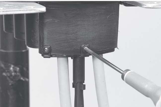
3.2.6 Install the metal bracket to the frame and secure with split pin. Secure the strength members. Install the spiral tube over the loose tubes.
