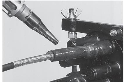
**11.11** Shrink down the end of the sleeve on the cable side. Heat till the sleeve shrinks down onto the cable and the green thermo-indicating paint is converted to black. A ring of red adhesive should be visible at the cable on the end of the sleeve.
