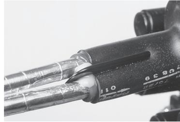
**6.7** Shrink down the end of the sleeve on the cable side. Heat until the sleeve shrinks down on the cables and take care that the green thermo-indicating paint is converted to black. Postheat the clip on both sides till the adhesive shows a proper flow on the clip between the two cables. Wait until the sleeve is cool to the touch before moving the cables.
