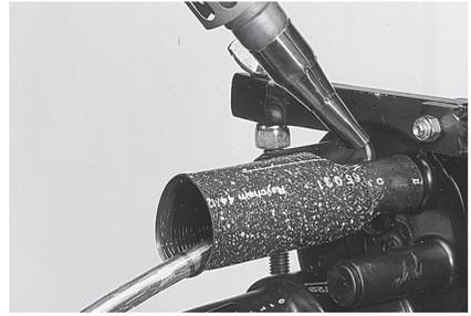
**11.10** Slide the cable seal over the port. Shrink the cable sleeve on the base side with the recommended hot air gun device. Use the reflector to ensure heat distribution around the outlet. Shrink sleeve until the green thermo-indicating paint is converted to black.
